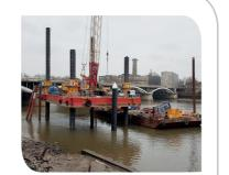
Red7Marine installs tubular driven piles in estuarine and near shore environments.
